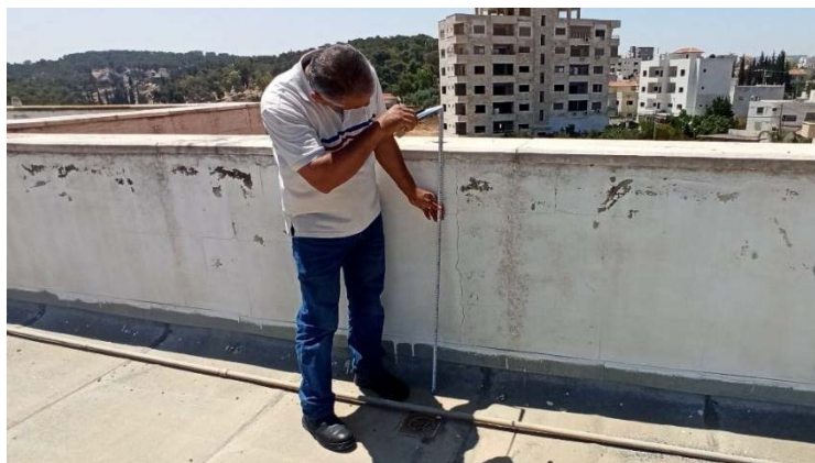
Figure 23. Parapet on the top of a school building
