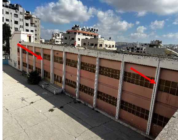
Figure 19. Formation of short columns in school buildings
