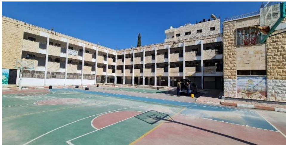
Figure 14. L-shaped school building
