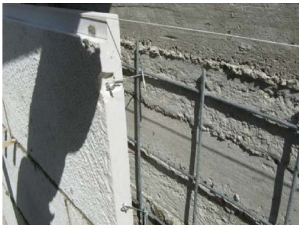
Figure 27. Fixation of stone cladding units to the masonry cement block exterior wall
