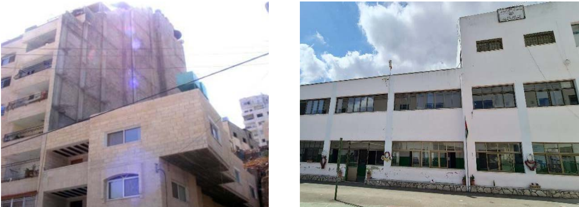
Figure 17. Buildings with setback vertical irregularities
