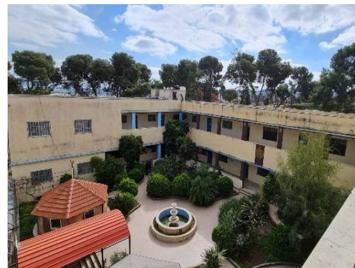
Figure 3. Concrete block exterior walls covered with plastering
