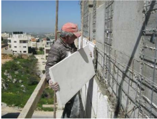
Figure 5. Stone cladding of a shear-wall building
