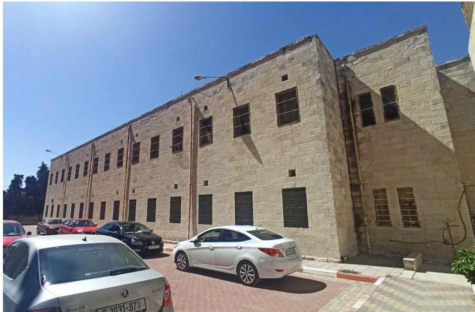
Figure 6. Masonry walls of a school building in Nablus city
