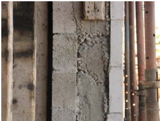
Figure 2. Masonry Walls, Concrete, Hollow block with Stone cladding
