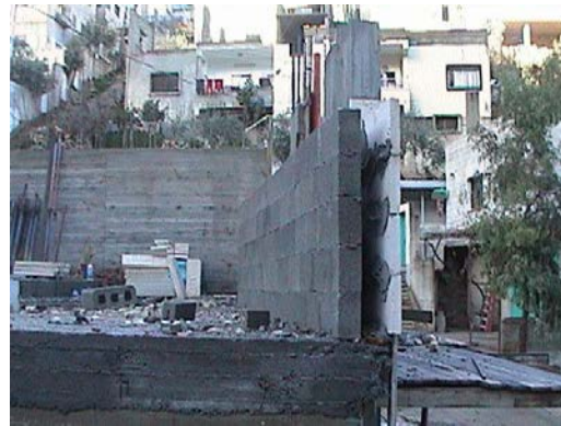
Figure 2. Masonry Walls, Concrete, Hollow block with Stone cladding
