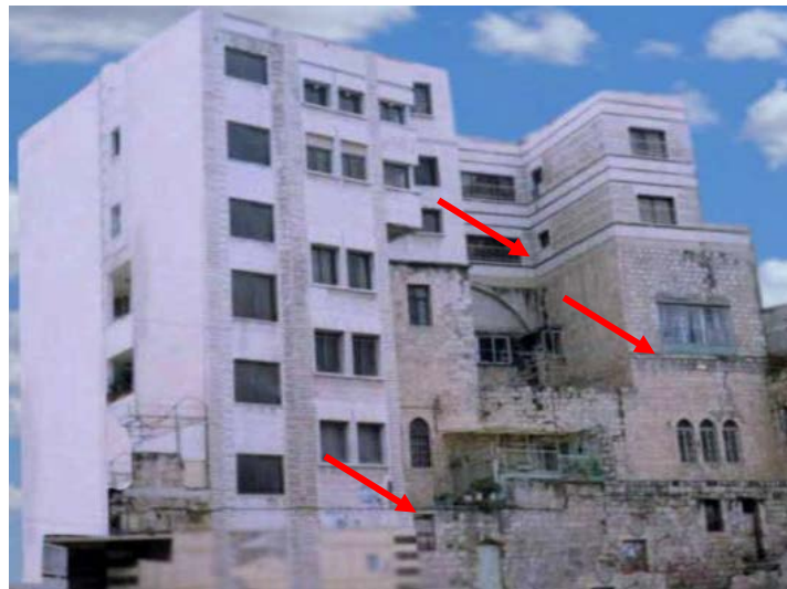
Figure 20. A building with different structural systems/materials across different floors
