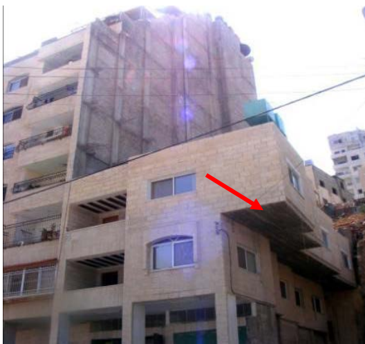
Figure 22. Buildings with long and heavily loaded cantilevers
