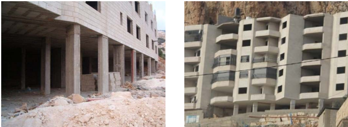
Figure 18. Buildings with soft (weak stories)
