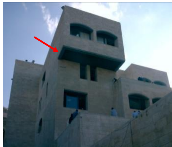
Figure 22. Buildings with long and heavily loaded cantilevers
