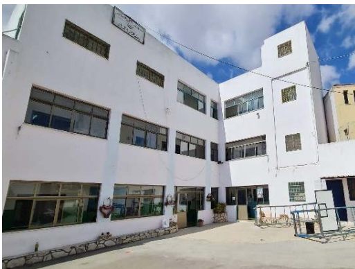
Figure 3. Concrete block exterior walls covered with plastering
