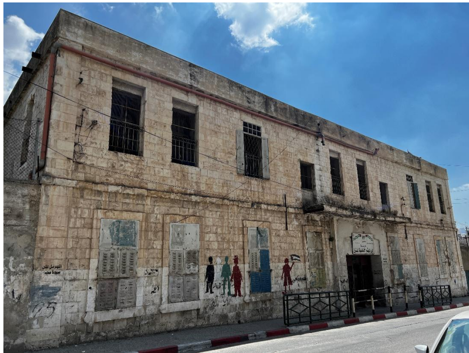
Figure 7. Masonry walls of a school building in Nablus city
