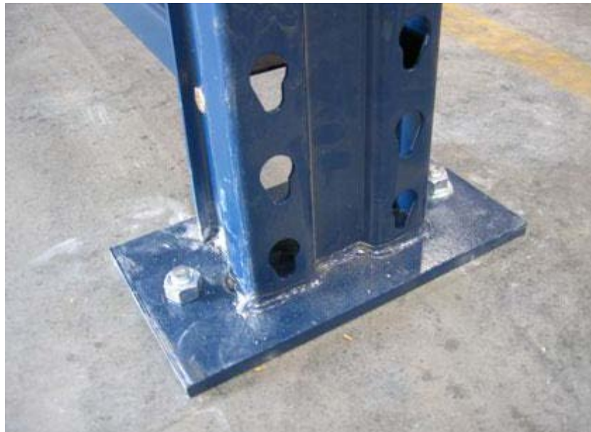
Figure 31. Fixing storage racks to the ground
