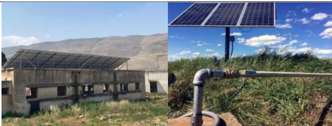
50 kWp Solar PV system for water pumping in the University Farm
