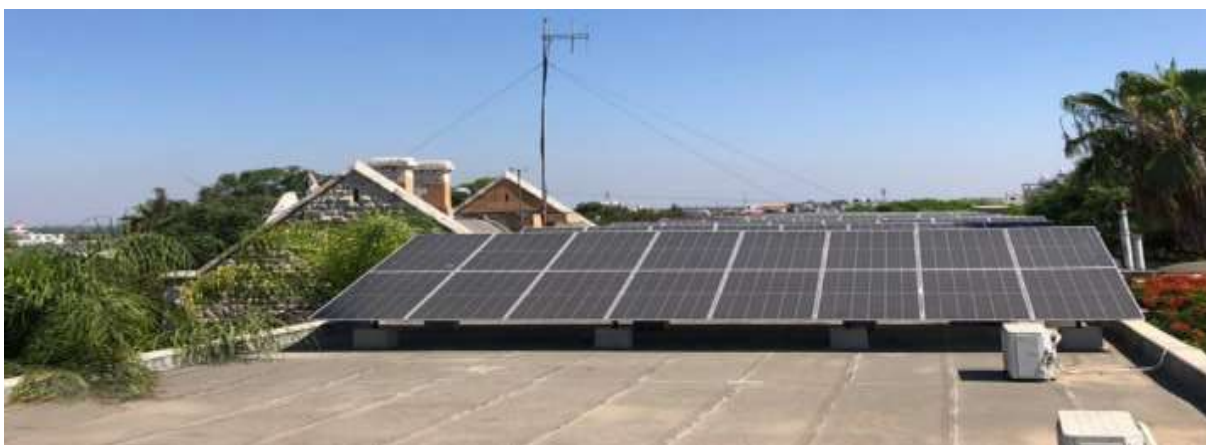
80 kWp Rooftop Solar Photovoltaic System at the Faculty of Agriculture and Veterinary Medicine building
