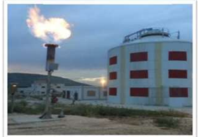
Digester tank in Nablus West WWTP with the gas flare
